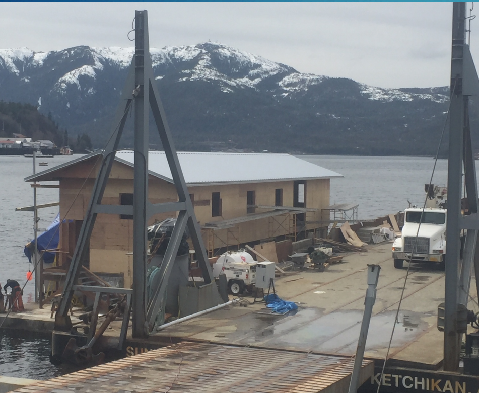
New Work Float
